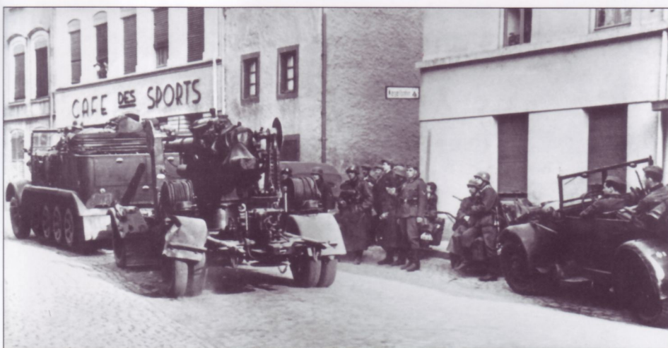
A mittlerer Zugkraftwagen 8-ton Sd.Kfz.7 tows an 8.8cm FlaK18 through a French town, quite probably during the campaign of 1940. The tractor has the KMm11 body style while the gun is identified as a FlaK18 by the Sd.Ah.201 limber units and the round leveling pads on the Kreuzlafette 18 (cruciform mount). At this period in time, the gun and tractor would have been "officially" finished in a two-tone camouflage scheme of Dunkelgrau RAL 7021 as a base color, over-sprayed with Dunkelbraun RAL 7017 in patches, so it covered roughly 1/3 of the item being painted.
