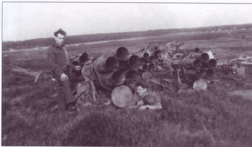
A pair of British/Commonwealth soldiers poses beside a heap of scrap that was at one time a battery of 21cm NbW42s; note that all have five launch tubes, which was a characteristic of this model. The round plate next to the man lying in the grass was designed to be lowered in front of the piece; this would raise the wheels off of the ground and along with the dug-in spades fitted to the end of the split trails, would steady it for firing.
