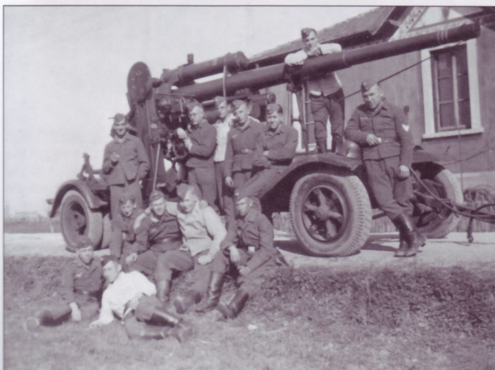
In an obvious display of camaraderie, this Luftwaffe crew poses with their veteran 8.8cm FlaK18; note the "kill rings", probably painted in yellow, near the gun tube's covered muzzle. There is also a gun-in-battery letter ("D") on the pneumatic recuperator cylinder, also probably in yellow. The round leveling pads identify the Kreuzlafette 18 (cruciform mount), while the single front wheels and fender configuration identify the limber as the Sd.Ah.201.
