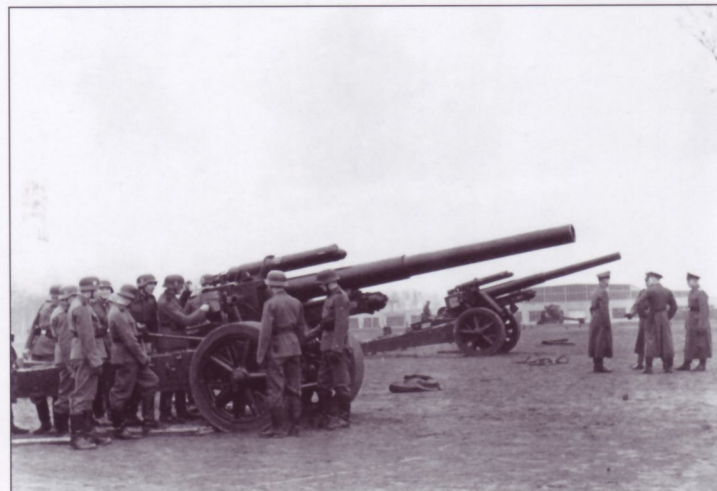
Obviously taken at a barracks or training facility, this 15cm s.FH18 is being closely inspected by a number of troops. Note that the near piece has the less-often-seen star pattern steel wheel hubs, with hard rubber rims, as does the other in the background. The link from the trail-mounted auxiliary elevation hand-crank (itself hidden by the troops) can be seen just below the elbow of the man manipulating the piece's breech block. In the far background is what appears to be a 10.5cm l.FH18.
