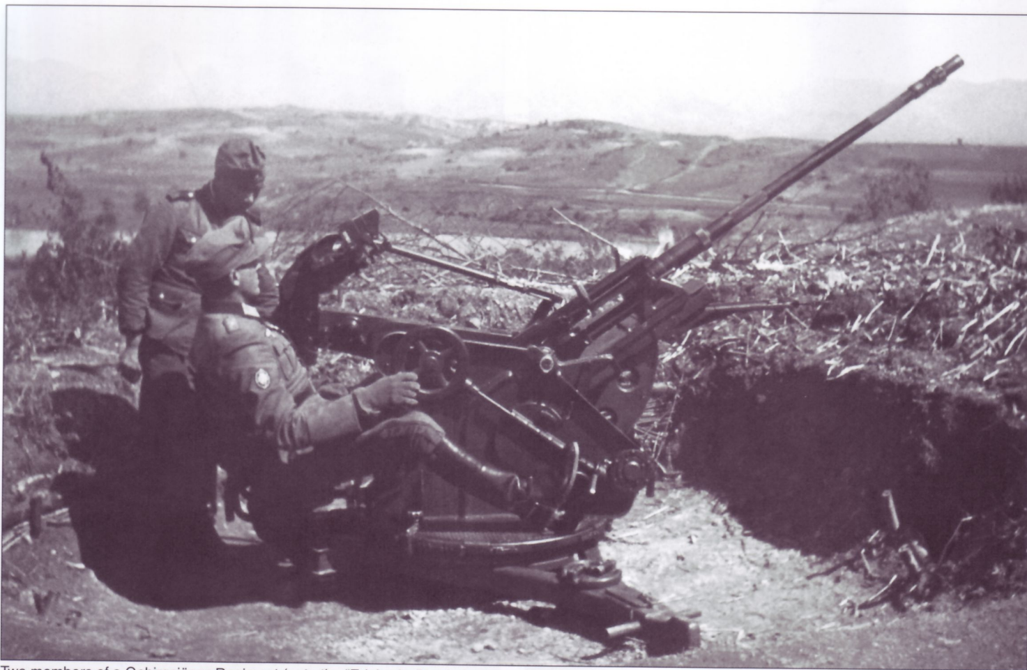
Two members of a Gebirgsjäger-Regiment (note the "Edelweiss" trade badge on the sleeve of the gunner) practice with their 2cm FlaK30. Two features of this gun are noticeable here: the unique style of muzzle flash suppressor and the centralized location of the gunner's seat. Both differed from those seen on the later 2cm FlaK38.
