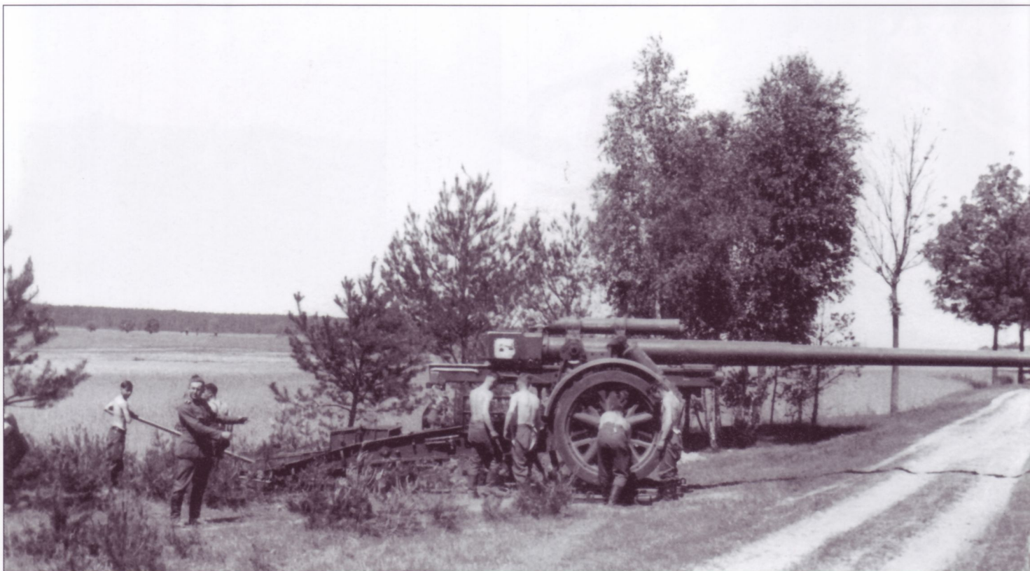
In an effort to create a single divisional heavy gun, Rheinmetall-Borsig developed the 15cm K18, beginning in 1933. This ordnance was hauled in multiple loads and when emplaced, was mounted on a two-piece platform that allowed full 360-degree traverse. A heavier and more cumbersome piece of ordnance, the 15cm K18 out-ranged the standard 15cm s.FH18, with an effective range of 24,500-meters vs. 13,325-meters.
