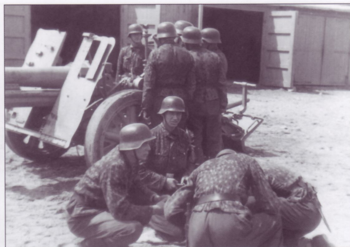
A group of what are apparently Waffen-SS troops receive instruction on various aspects of the 15cm s.IG33 heavy infantry gun. Although much of the gun is obscured, the configuration of the shields as well as the small flap that covered the gunner's sight can be readily seen, as can the "T"-shaped handle at the end of the box trails that was used to move the piece. Note also how the gunner's sight could be (if conditions warranted it) telescoped upwards to clear the top of the shields.
